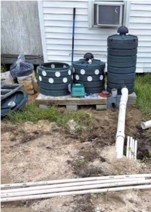
▲ The Anua Puralinity pH Biobuffer set and ready to be plumbed (far right).
