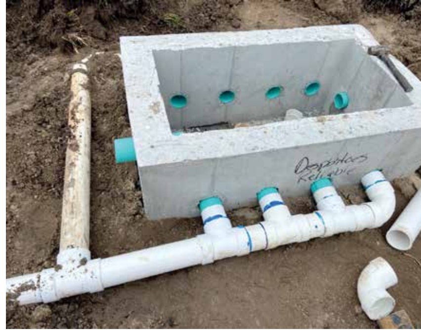
▼ The distribution box during plumbing.
