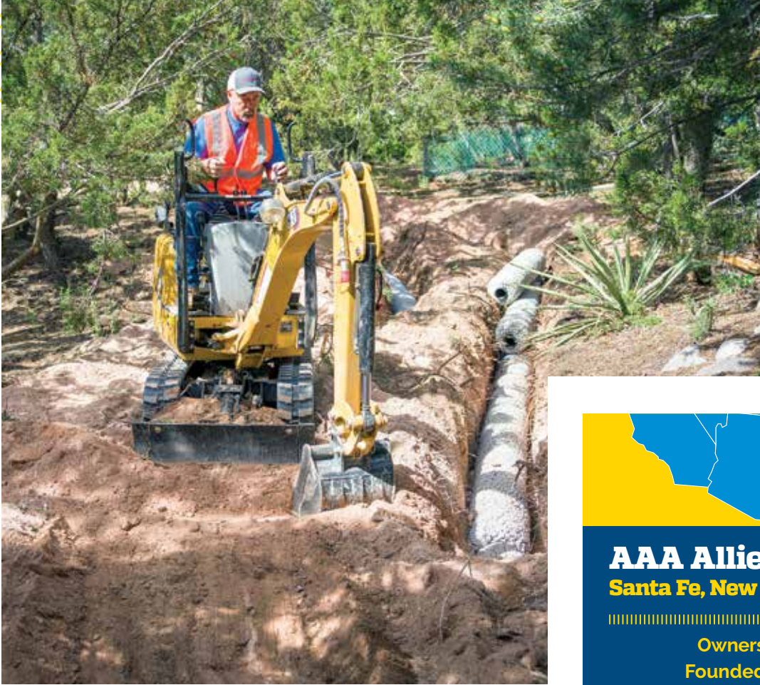
◀◀ Ralph Dotson digs a trench using a Caterpillar 300.9 mini-excavator.
