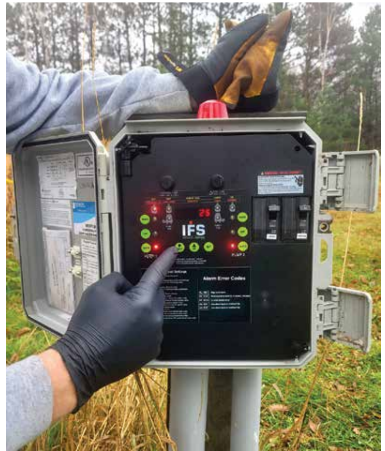
▲ An example of a flow equalization panel from SJE Rhombus that can be helpful at monitoring and adjusting flow in vacation rental home onsite systems. (Photos courtesy of Sara Heger)
