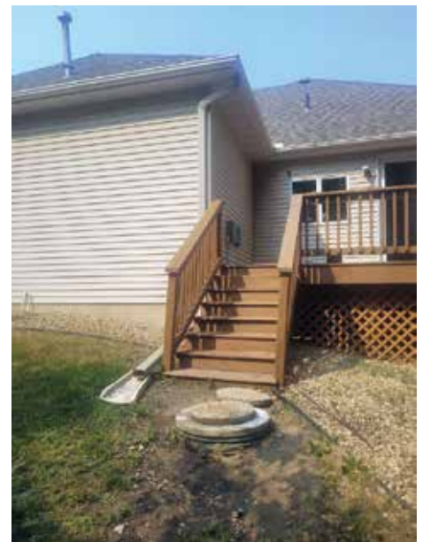
Small lots sometimes leave system designers or installers little choice over where to place treatment system components, such as placing a tank access close to deck stairs or use up much of the backyard for a mound. (Photos provided by Sara Heger)
