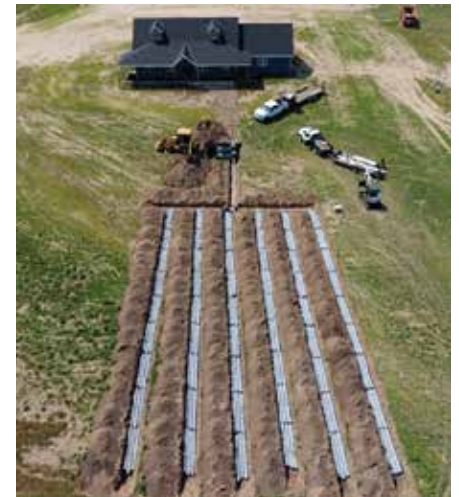
⚡ This aerial photo showing the installation of an EZFlow system installation is included in homeowner training materials at the NOWRA website. (Photos and graphics courtesy of the National Onsite Wastewater Recycling Association)
