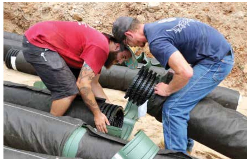
▼ Isaiah Muldoon, left, and Kevin Phipps, right, of BBB Septic in Bentonville, Arkansas, join two sections of AES pipe during the installation.
