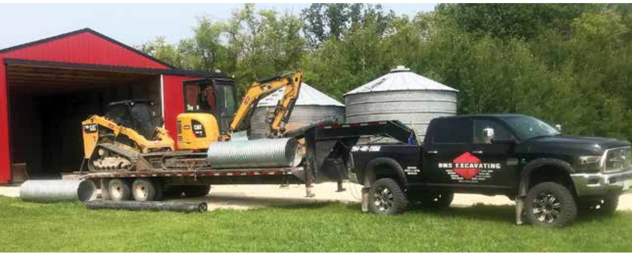
◀◀ A 2012 Ram 3500 is pulling a Caterpillar 279 skid-steer and Caterpillar 303.5 excavator heading out to an installation. (Photos courtesy of BNS Excavating)
