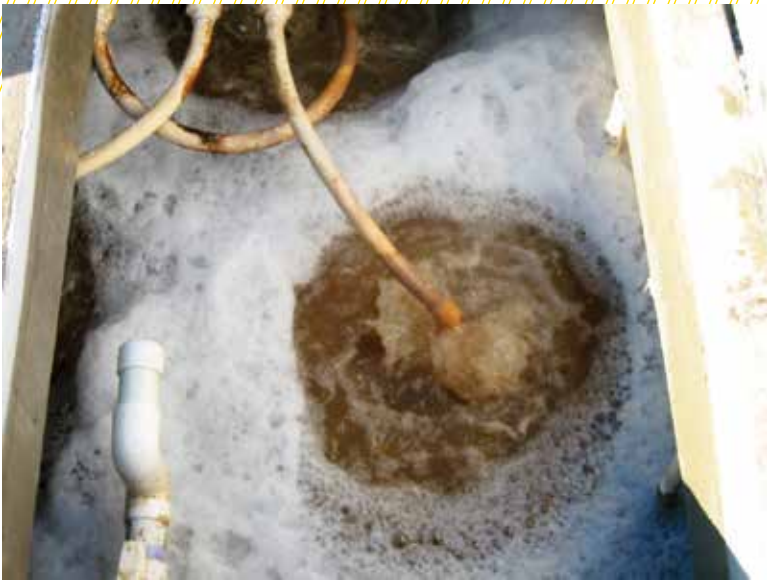
▲ A BioMicrobics ATU with a blower pushes air into the airlift, producing recirculation of oxygenated water throughout the submerged media.
