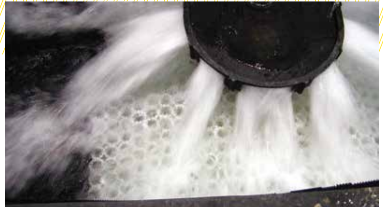
▲ A BioMicrobics ATU with a blower pushes air into the airlift, producing recirculation of oxygenated water throughout the submerged media.
