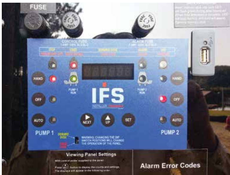
▲ A closeup look at the interface of an Installer Friendly Series of dosing system by SJE Rhombus. (Photos provided by Sara Heger)
